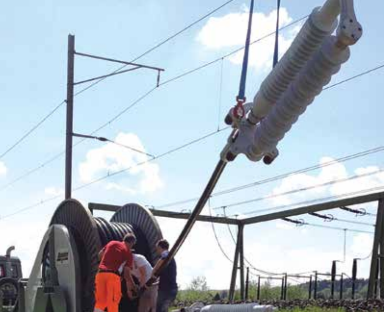
Movable preassembled energy back-up solutions for easy and quick installation to bypass transmission lines.
