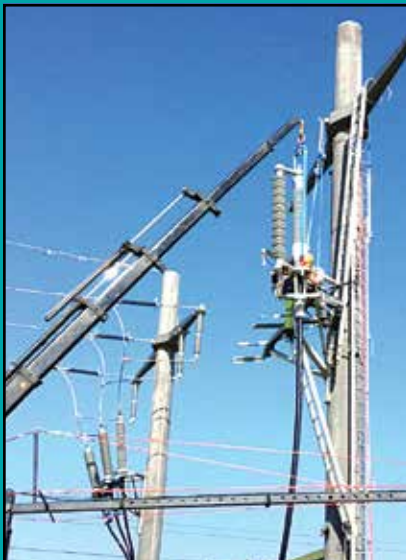
New dry type terminations lifted onto tower for final installation.
